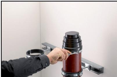
1. Slide the open end of the OHA Multi-Connector over the end of the tube and position the hose clamp in the recess provided. Then tighten the hose clamp firmly while maintaining its position.
